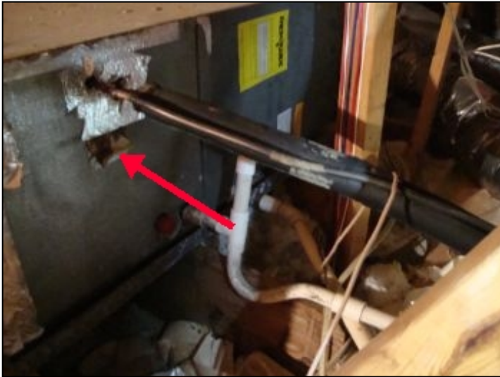
Air leaking on secondary A/C attic unit
