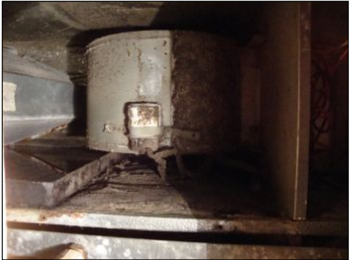
Recommend A/C in attic be serviced and cleaned
